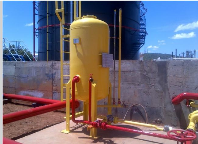
Angus Bag Tank Modules are designed for use with the BPP range of proportioners to balance the foam concentrate supply with the fire main water pressure at the inlet..
