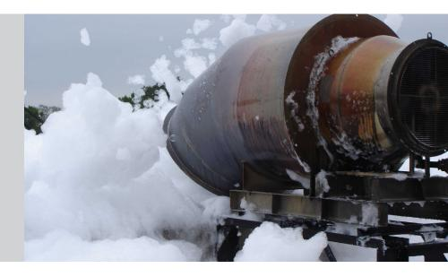
High expansion foam systems represent the most effective protection for LNG (Liquefied Natural Gas) spills, both for vapour reduction and dispersion as well as for radiant heat reduction and fire control.
